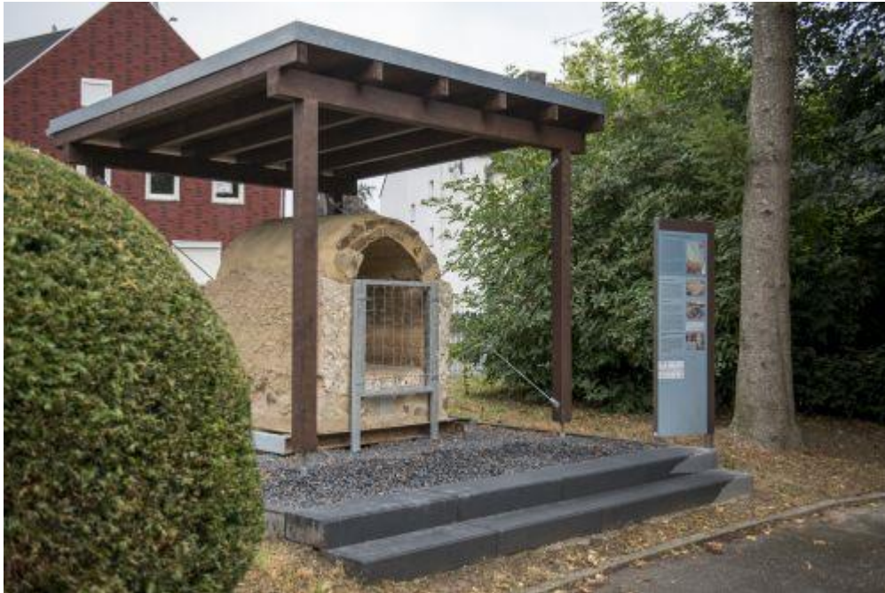
Figure 7: Final re-installation of a section of the Roman water pipeline with canopy and information panel at the Heilig-Geist-Gymnasium in Würselen. (M. Zanjani/LVR-State Service for Archaeological Heritage)
