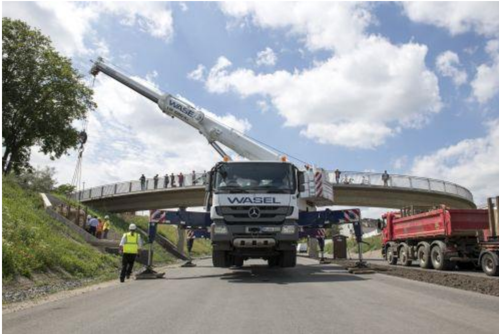
Figure 4: Placing a segment of the Roman water pipeline close to its find spot in the embankment of the new road. (M. Zanjani/LVR-State Service for Archaeological Heritage)
