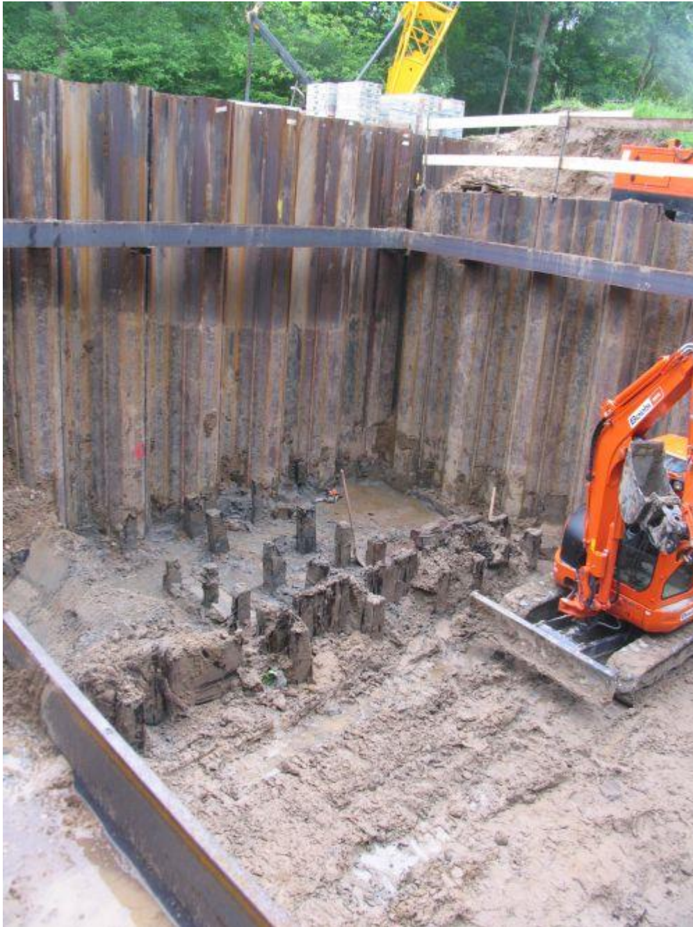
Figure 5: Wooden grate of an older structure in the area of the Rhine dyke near Biblis-Nordheim (Photo: R. Klausmann, hessenARCHÄOLOGIE, Darmstadt field office)
