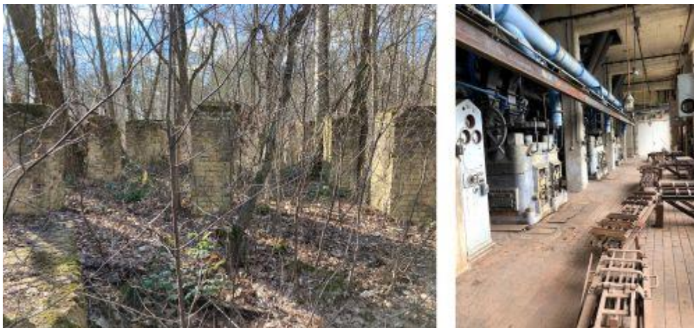
Figure 14: Left: Foundations of the loading plant at the Caroline I lignite mine (1890-1913) near Weißwasser/O.L.; Right: Briquette presses in the Werminghoff briquette factory (Photos: A. Prust, Saxon State Office for Archaeology)
