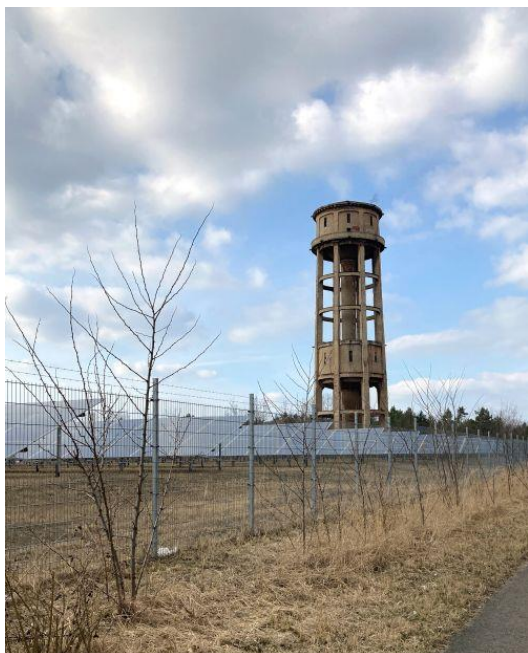
Figure 15: Water tower Lautawerk, 2022 (Photo: M. Neubacher, Saxon State Office for Monument Preservation)
