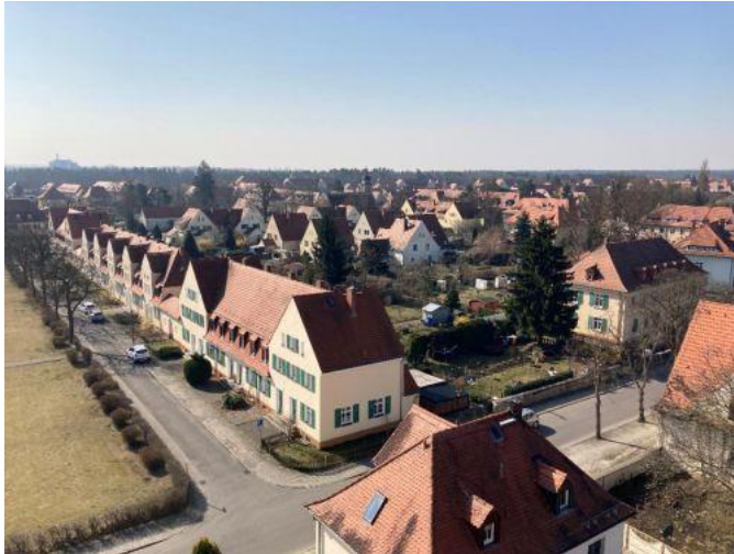
Figure 8: District Lauta-Nord, 2022 (Photo: M. Neubacher, Saxon State Office for Monument Preservation)
