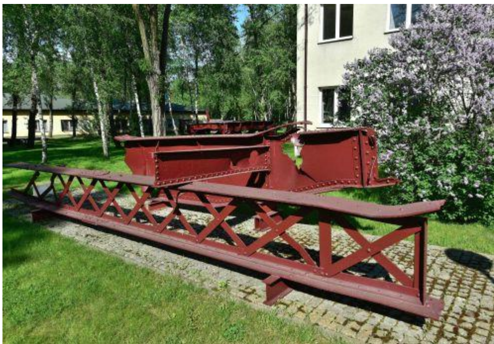
Figure 6: Fragment of the Kierbedź Bridge - the first steel bridge over the Vistula River in Warsaw built in 1859-1864 - presented near the Road and Bridge Research Institute in Warsaw. © Adrian Grycuk, 2017, CC BY-SA 3.0 PL
