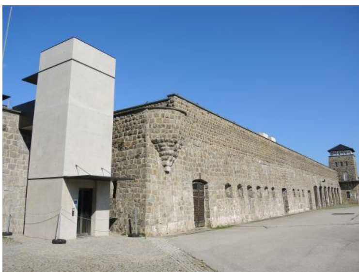
Figure 2: The elevator built in 2018 at Mauthausen memorial, Austria (Image credit: G. Carr)
