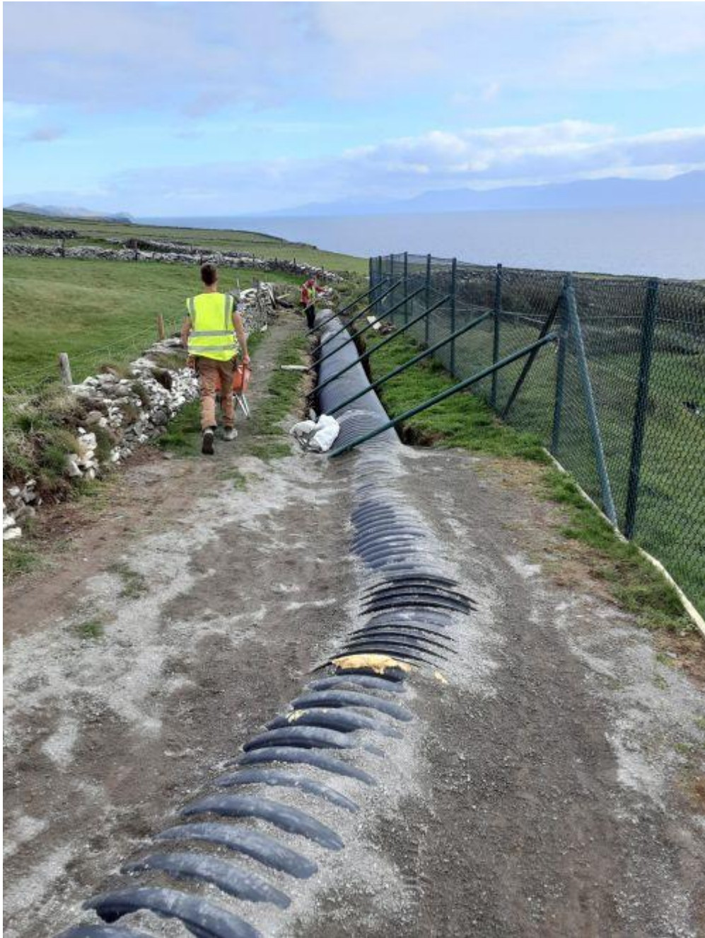
Figure 9: New culvert drainage pipework (Image credit: OPW)
