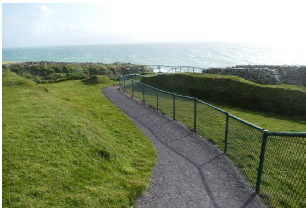
Figure 7: New safety fencing installed in 2019 by OPW to allow safe access to the site for visitors (Image credit: OPW)
