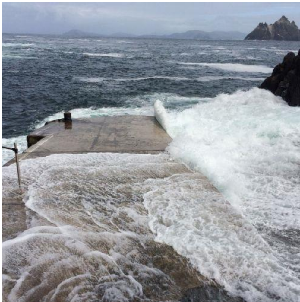
Figure 20: Landing pier during high sea swells (Image credit: OPW)
