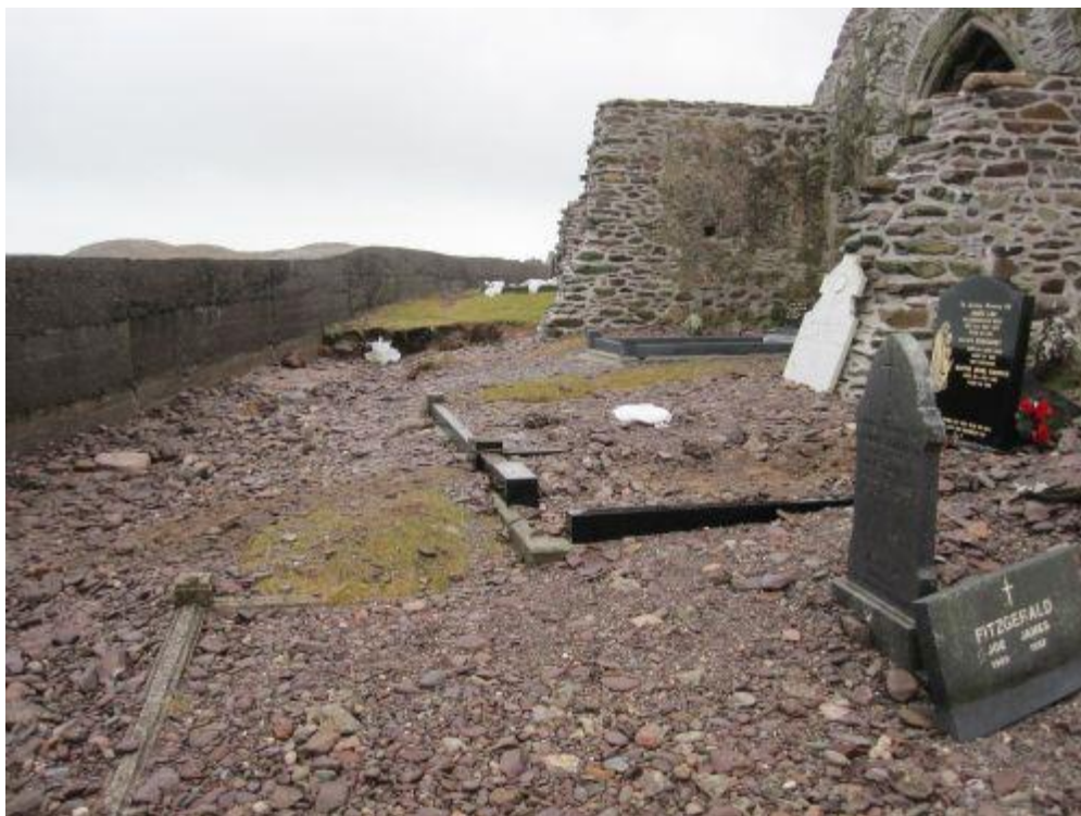
Figure 24: Storm damage in 2014 (Image credit: OPW)
