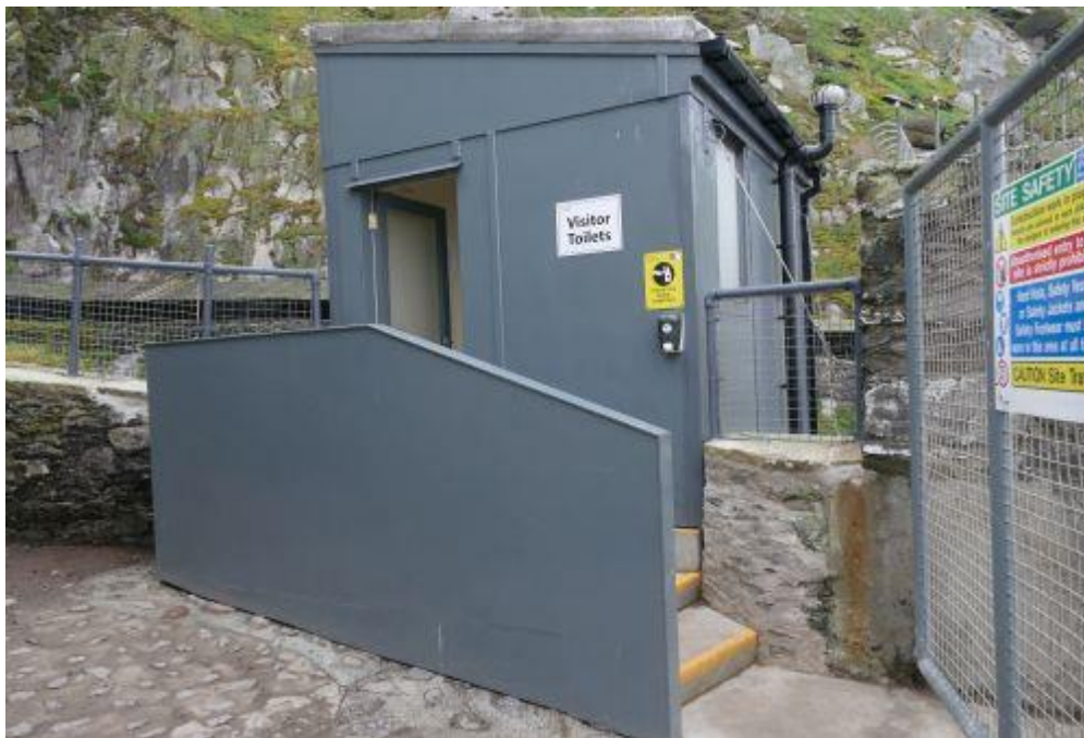
Figure 21: New visitors' toilets installed near the helipad in the 2021 season (Image credit: OPW)
