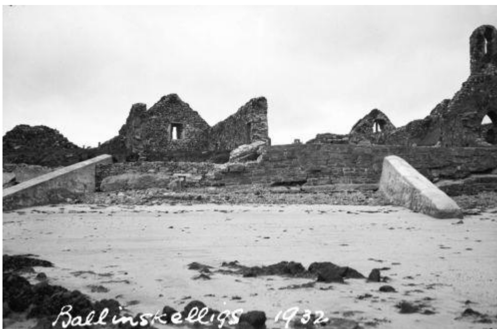
Figure 27: Archive image of the former sea wall from 1932 (Image credit: OPW)
