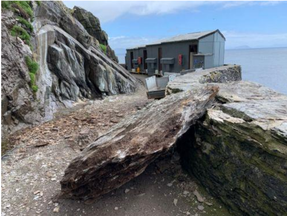
Figure 16: Rock fall in 2020 (Image credit: OPW)
