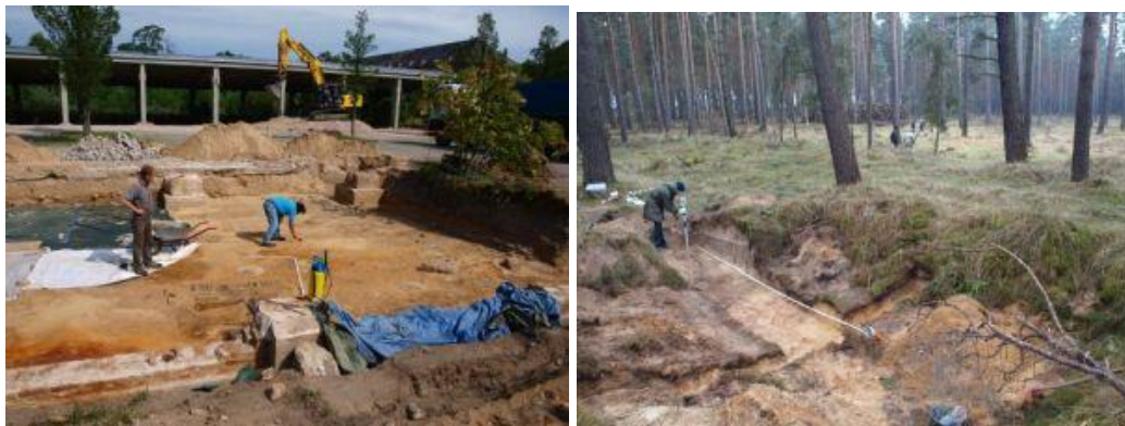
Figure 11 (left): Excavation of the remains of a mosque in the WWI 'Half Moon Camp' under Wehrmacht halls in Wünsdorf (Photo author)
