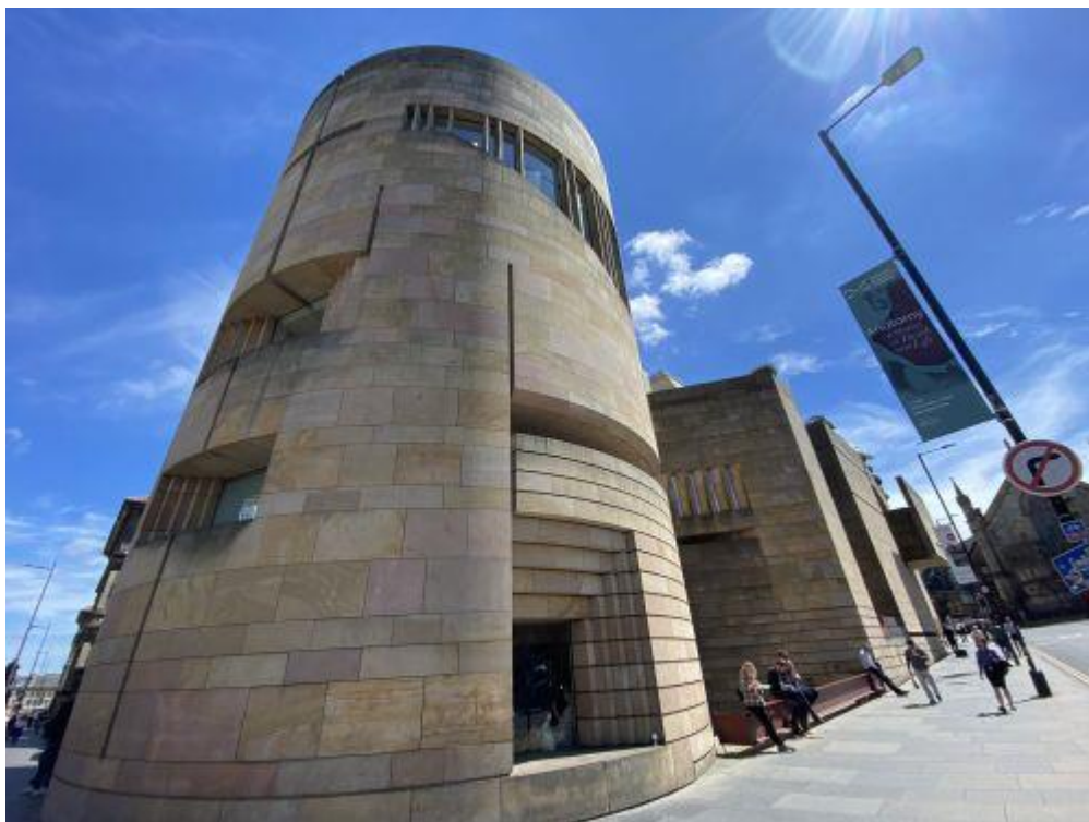
Figure 7: The exterior of the new National Museum of Scotland building, faced with Scottish Clashach stone, designed as an allusion to medieval fortifications. Image credit: W. Givens
